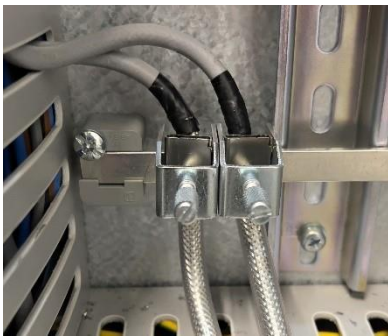
Figure 15: Cable connection terminals for control cabinet mounting
