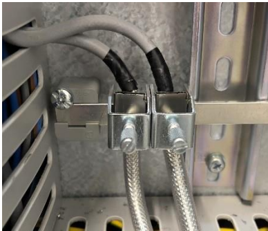
Figure 6: Cable connection terminals for control cabinet mounting
