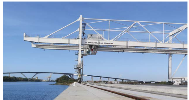
在 RMG 的起升装置上安装 MAG Installation of the MAG at the crane hoist of a RMG crane
