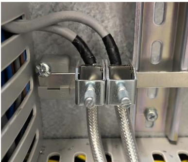
Figure 15: Cable connection terminals for control cabinet mounting
