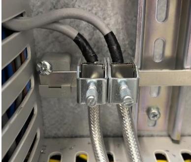
Figure 6: Cable connection terminals for control cabinet mounting
