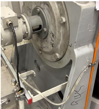
Figure 12: Connecting the grounding strap to an earthing point
